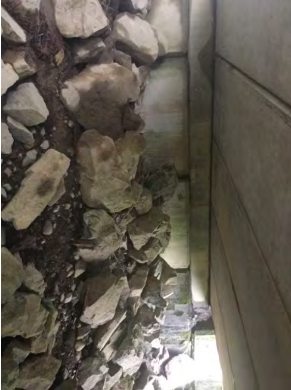
Right Bank Abutment when facing downstream
