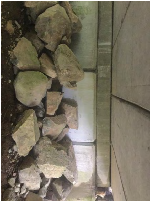
Left Bank Abutment when facing downstream
